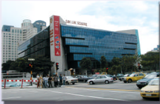
Sim Lim Tower Car Park – Sim Lim Square, Rochor Canal Road Singapore 2 Entry 2 Exit Lanes Season Parking only
